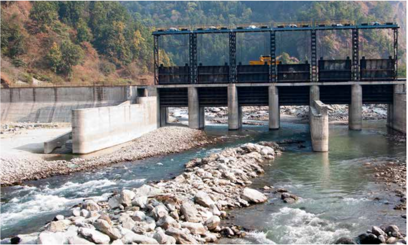
Kabela B-1 Hydroelectric project (intake section) on the Kabela river between Thumberding and Tharpu, Taplejung & Panchar District, Nepal. © Marc Boettcher/Alamy Stock Photo
